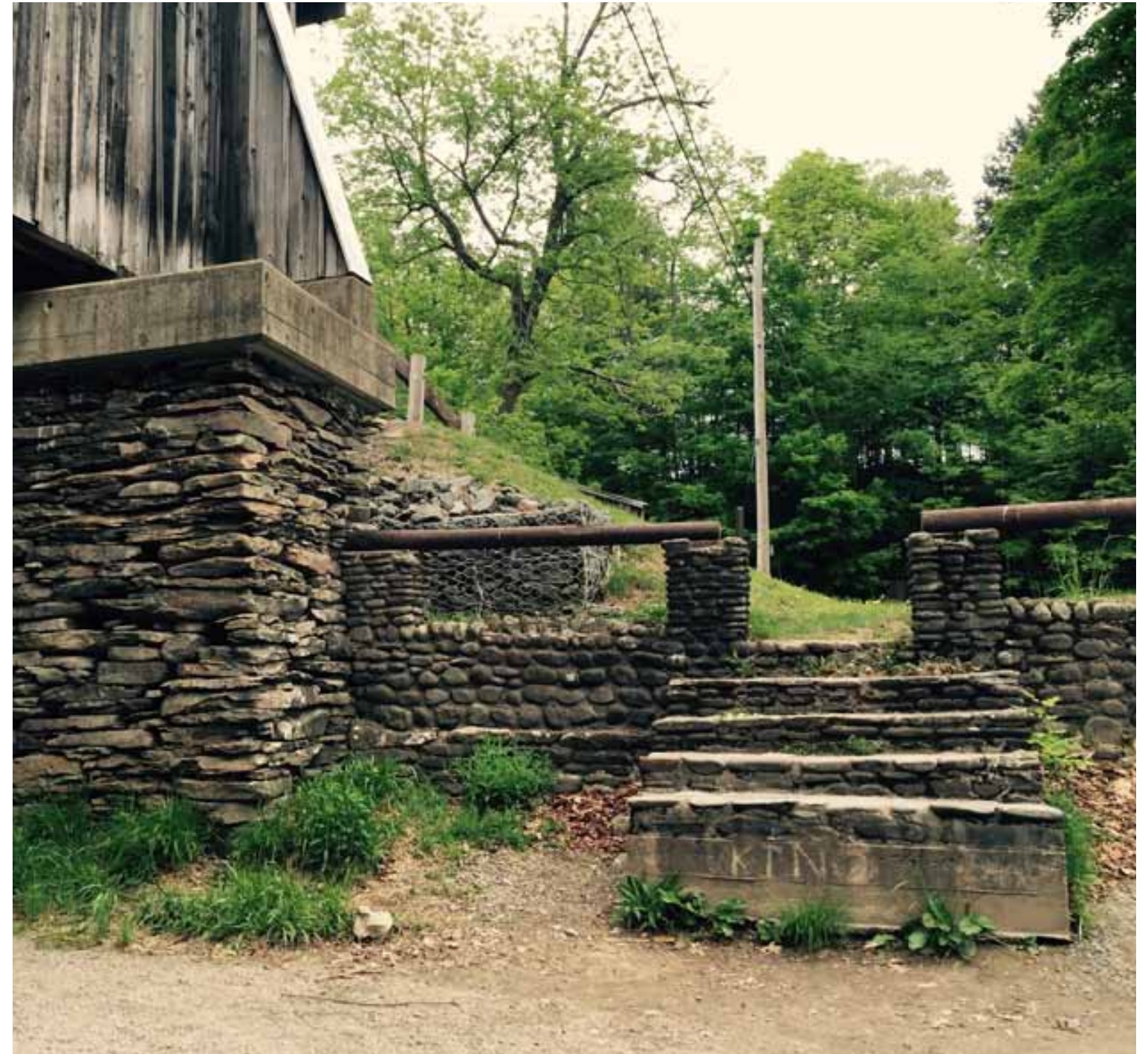
STONE WALLS AND RAILINGS ON BOTH SIDES OF THE BRIDGE WERE BUILT BY THE CCC IN THE 1930S
