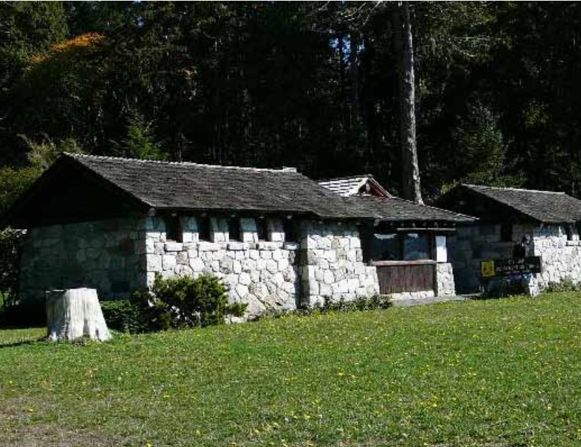
CCC INTERPRETIVE CENTER PRECEDENT, DECEPTION PASS, WA
