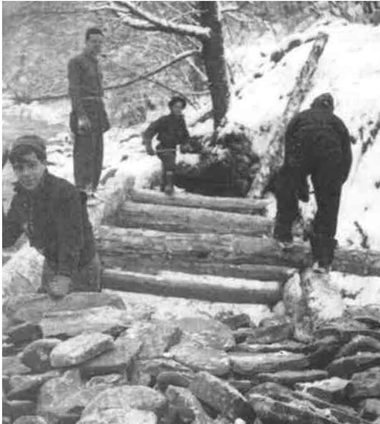
CCC MEMBERS BUILDING BEAVERKILL'S SIGNATURE STONE WALLS
